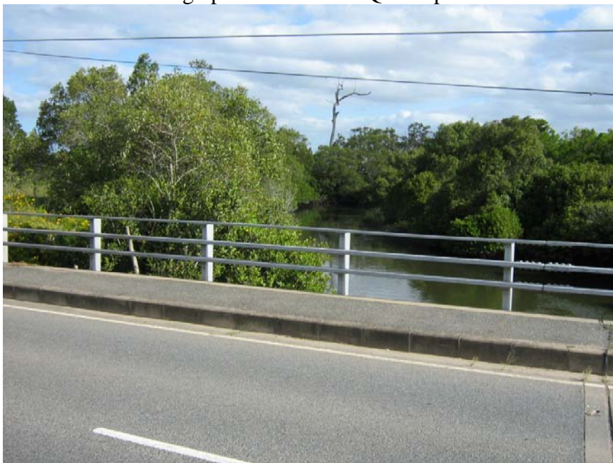
Looking upstream towards Wynnum Road from bridge
