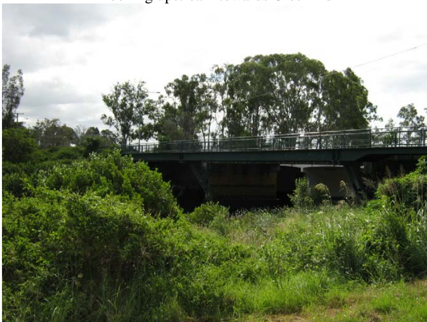
Looking downstream towards Murarrie Rd
