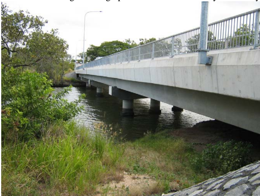
Looking upstream towards Gateway Motorway
