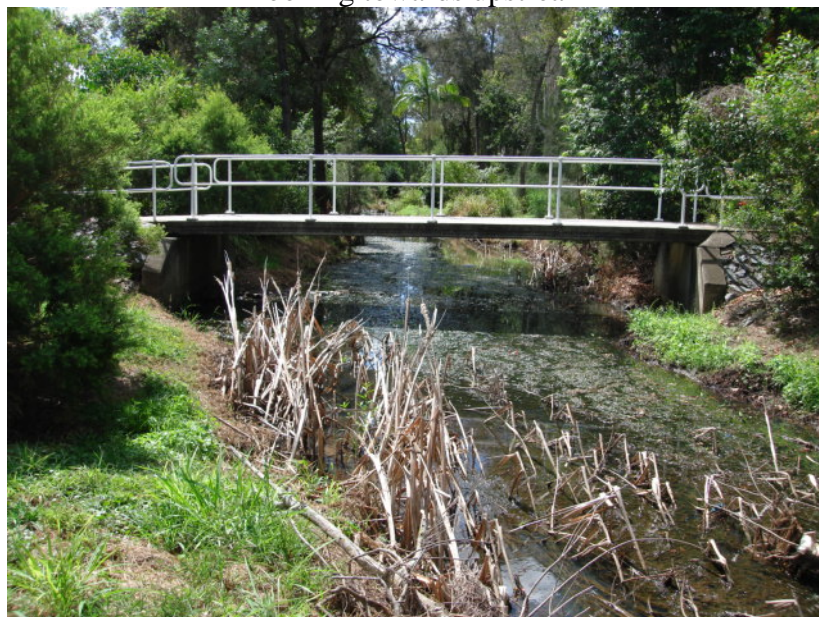
Looking towards downstream
