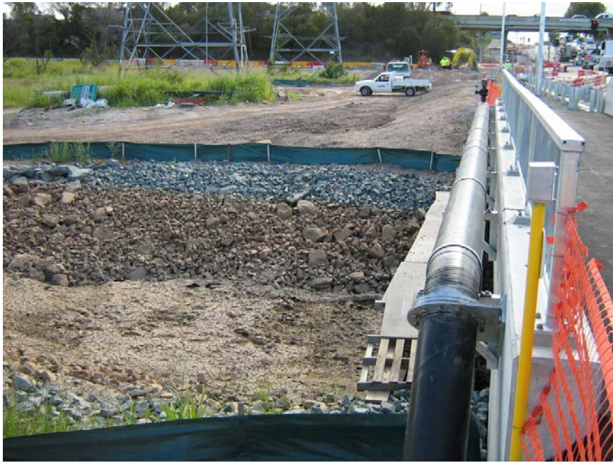
Looking downstream towards Gateway Mwy
