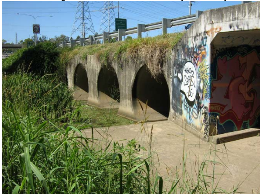
Looking upstream towards Gateway Motorway
