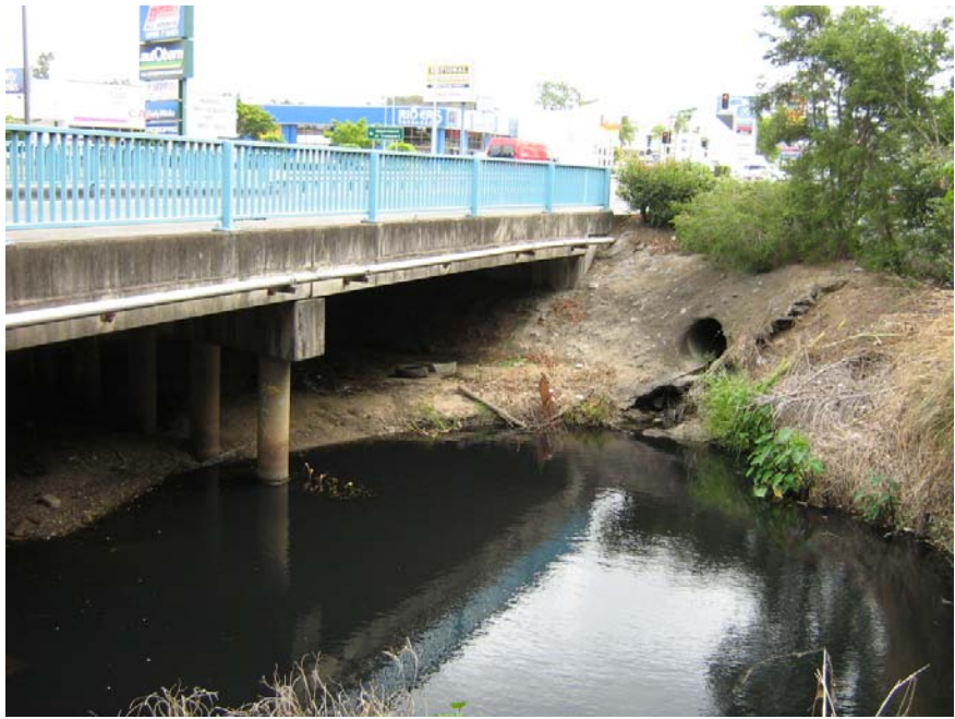
Kessels Road Bridge looking from downstream
