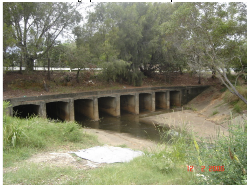
Looking downstream towards Beenleigh Rd
