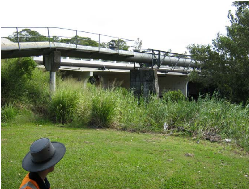
Looking upstream towards Creek Rd
