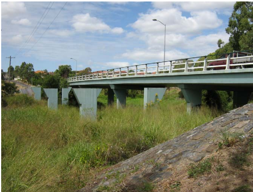
Looking upstream towards Gateway Motorway
