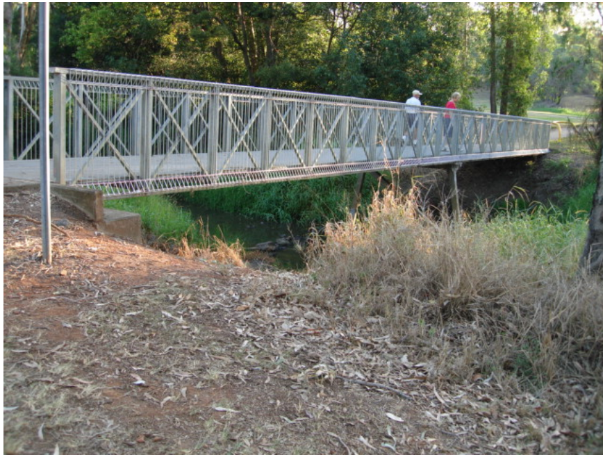
Looking downstream towards Eromanga St
