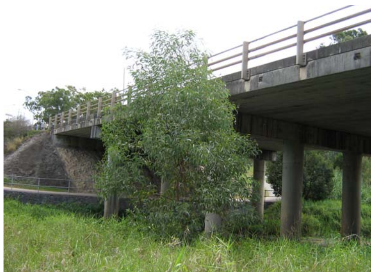
Looking downstream towards Ham Road
