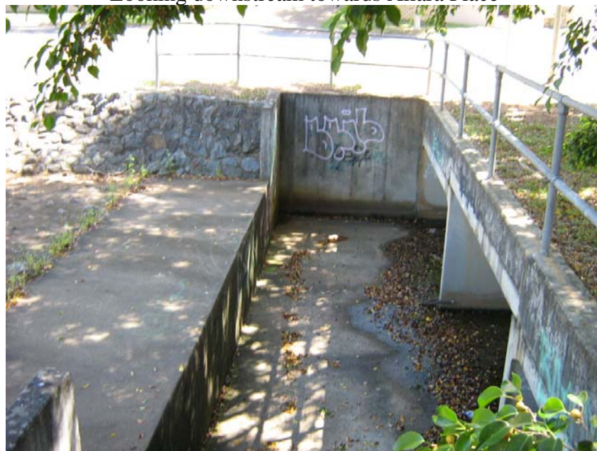
Looking downstream – drop structure
