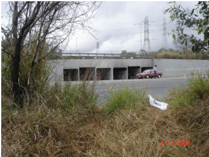
Looking downstream towards Creek Road
