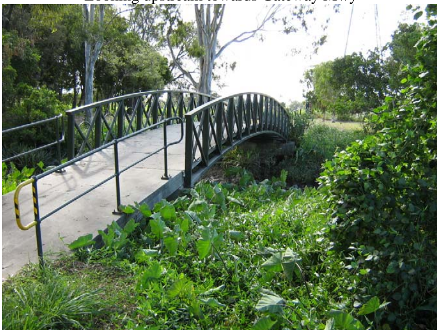
Looking downstream towards Wynnum Rd
