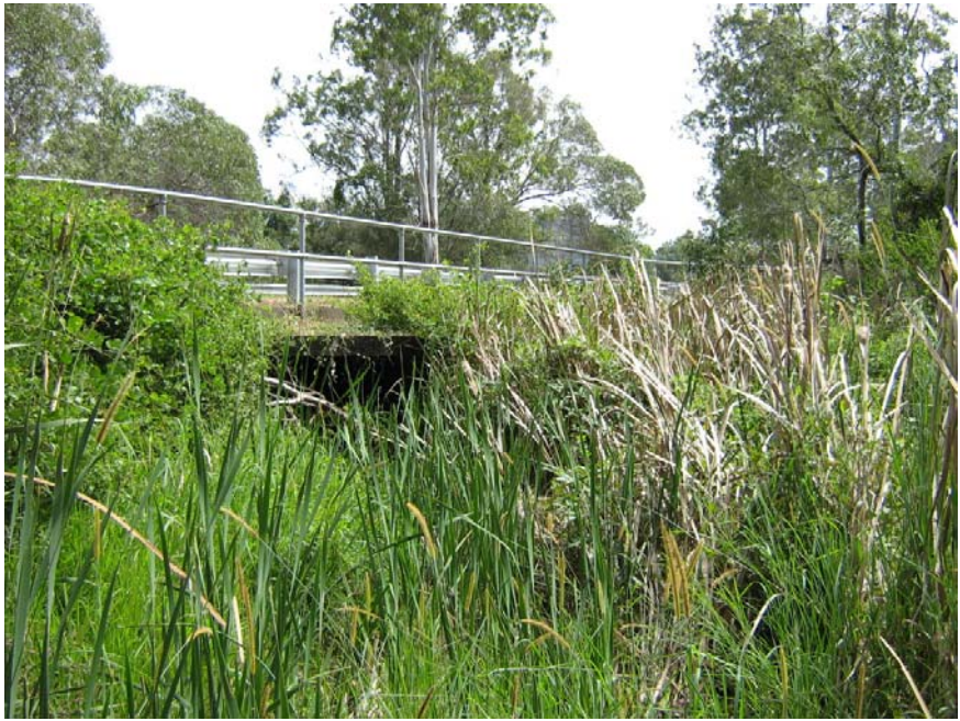
Looking downstream towards South East Freeway
