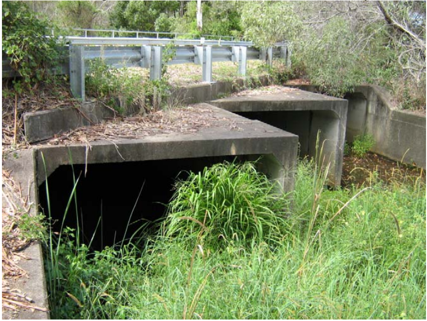
Looking upstream towards Priestdale Road
