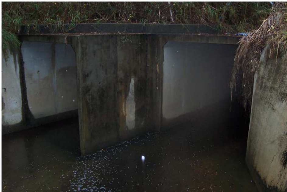
Looking upstream towards Padstow Rd
