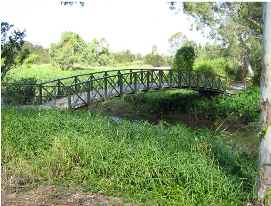
Looking upstream towards Gateway Mwy
