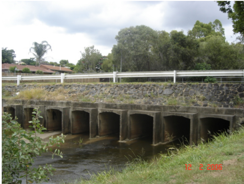
Looking upstream towards Compton Rd
