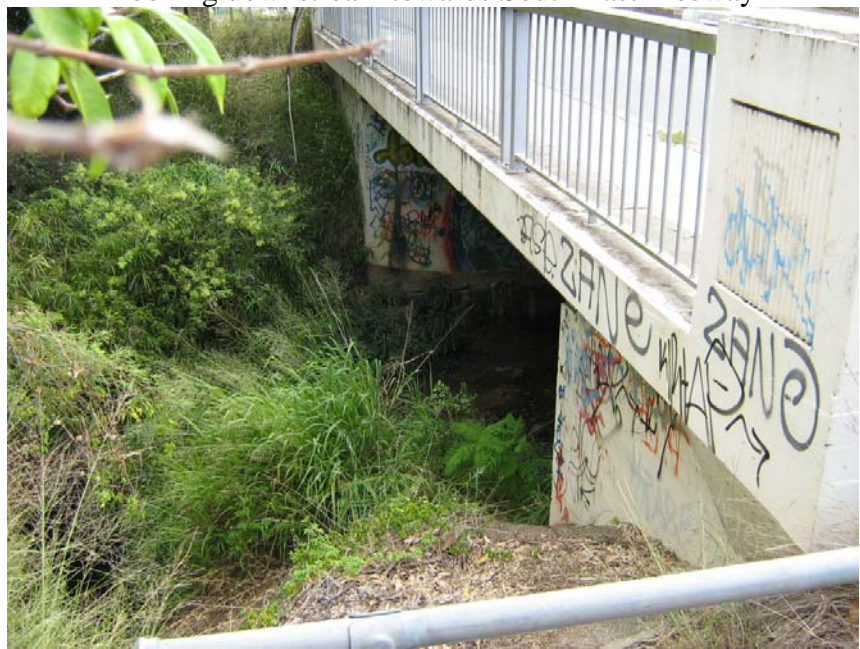
Looking upstream towards Klumpp Road
