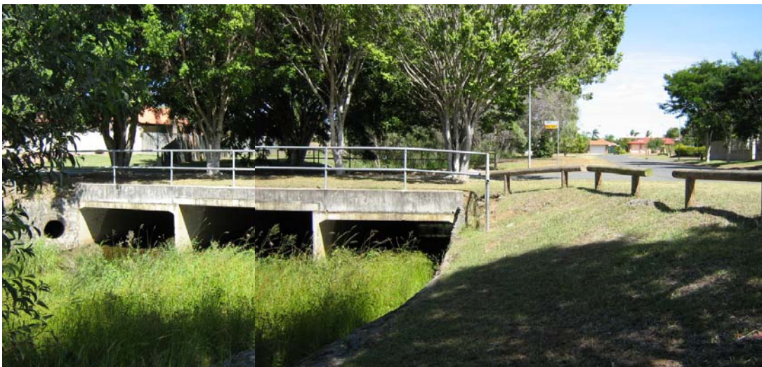
Looking upstream towards Bordeaux Street
