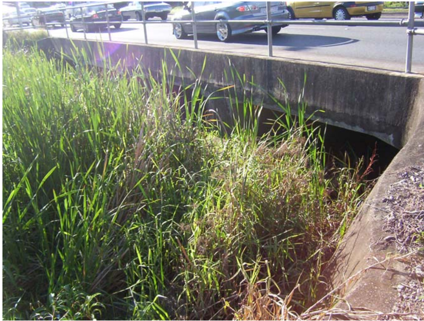
Looking downstream towards Altandi St
