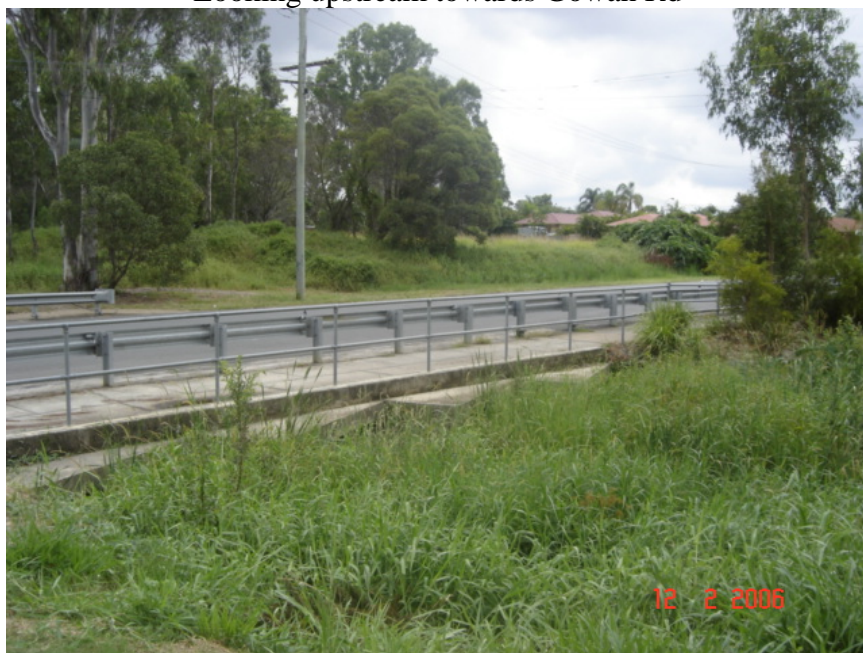
Looking downstream towards Beenleigh Rd
