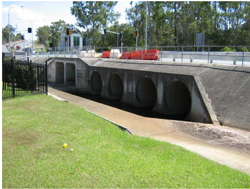
Looking downstream towards Brandl Street
