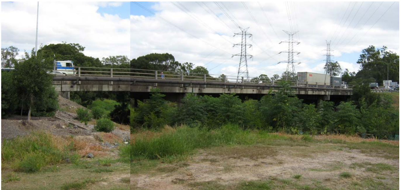
Looking upstream towards Stackpole Street
