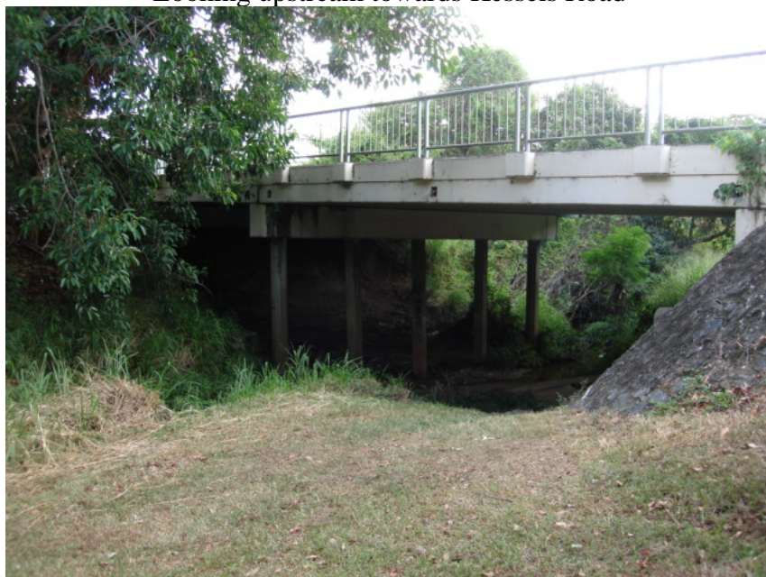
Looking downstream towards Padstow Road
