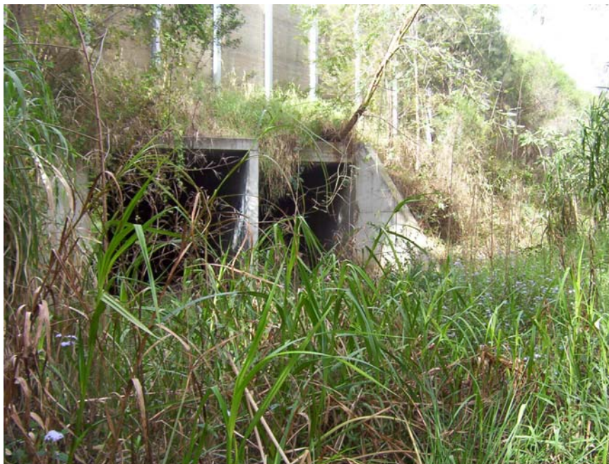
Logan Road culvert in Garden City branch: looking from upstream
