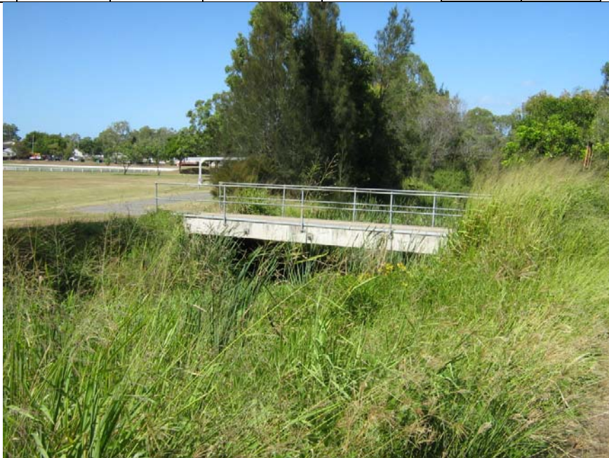
Looking upstream towards Beenleigh Rd
