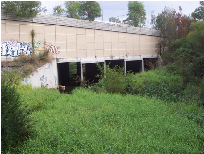
Looking upstream towards Padstow Rd
