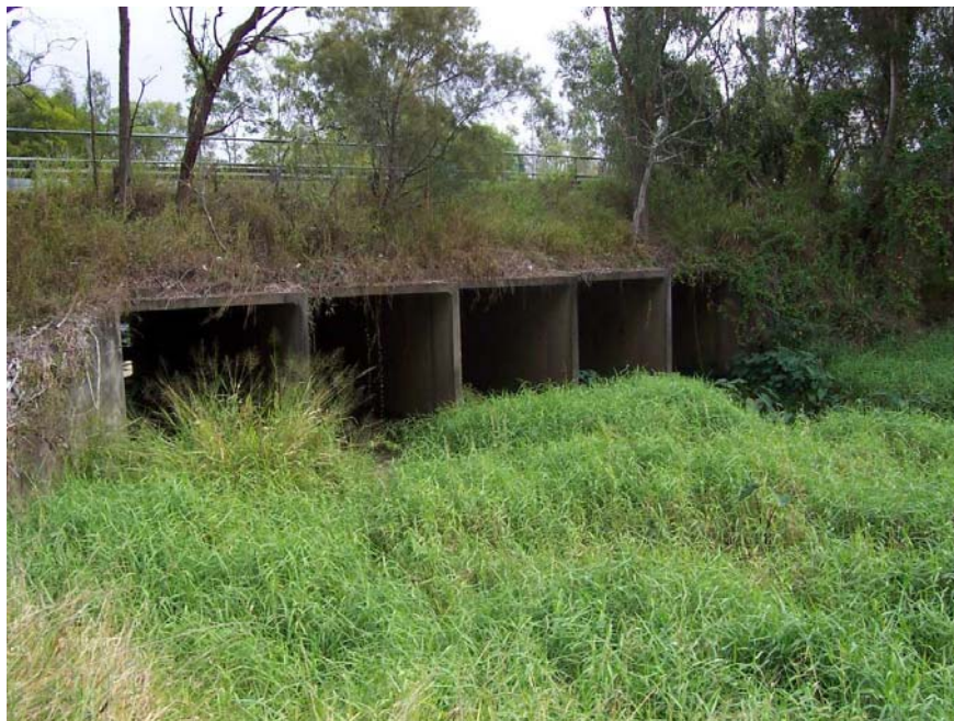
Looking downstream towards Kavanagh Rd
