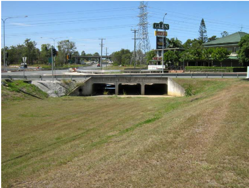
Looking upstream towards Gateway Motorway
