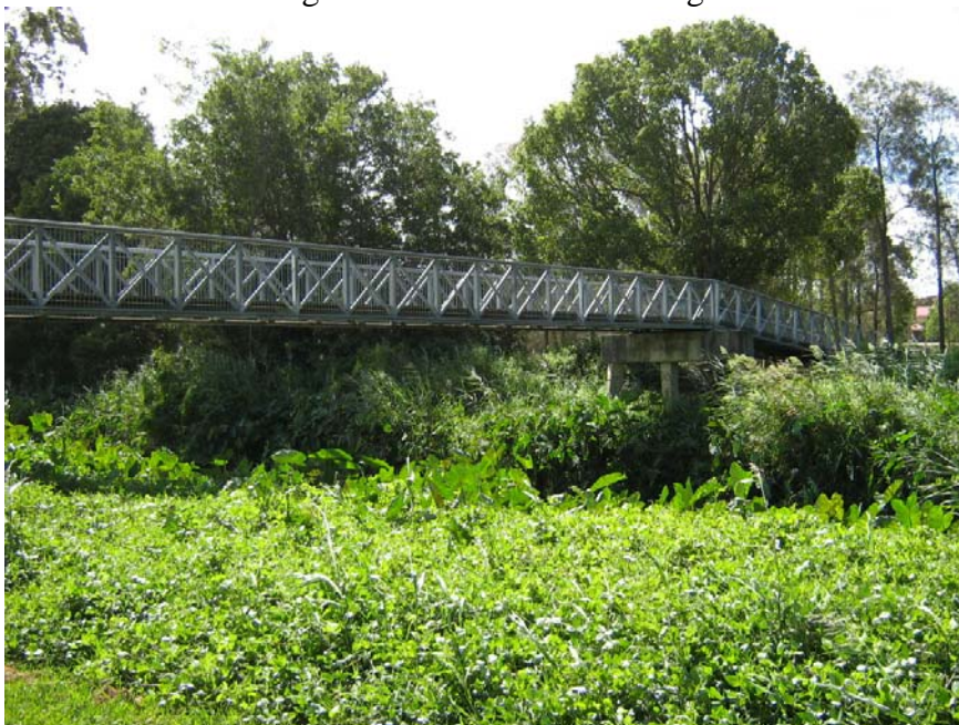
Looking upstream towards Meadowlands Rd
