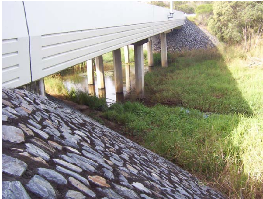
Looking upstream towards Miles Platting Road
