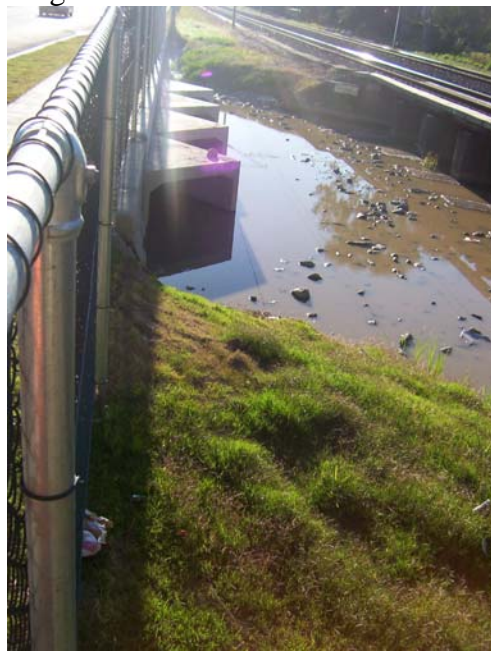
Looking upstream towards Perse Rd
