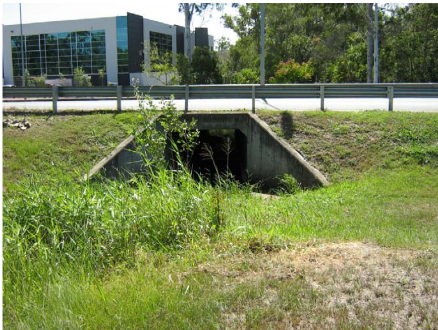
Looking downstream towards South-East Freeway
