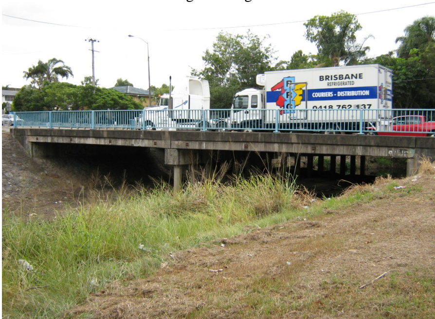
Kessels Road bridge Looking from upstream
