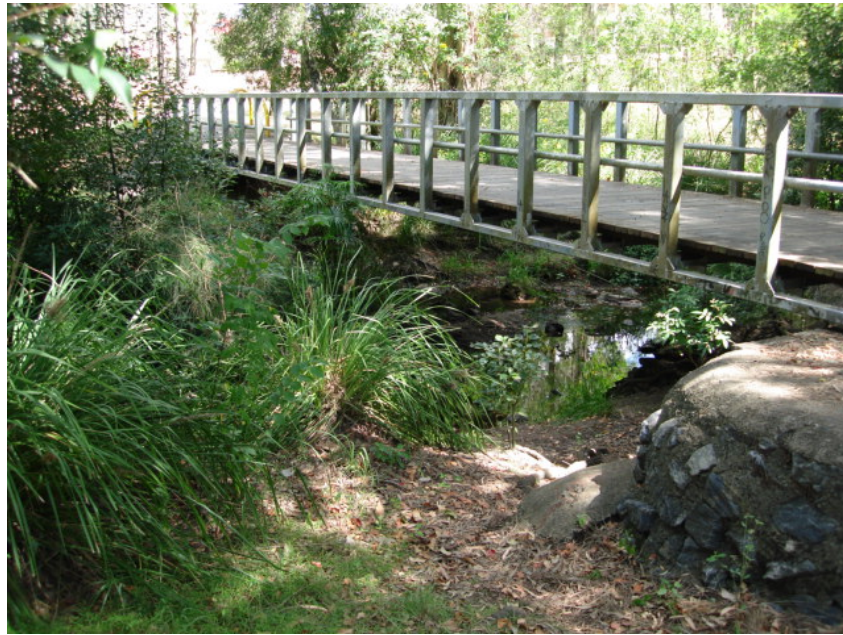
Looking from downstream of the Bridge
