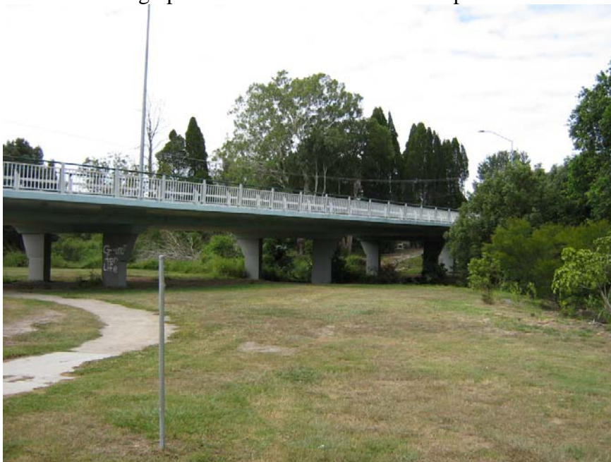
Looking downstream towards Pine Mountain Rd
