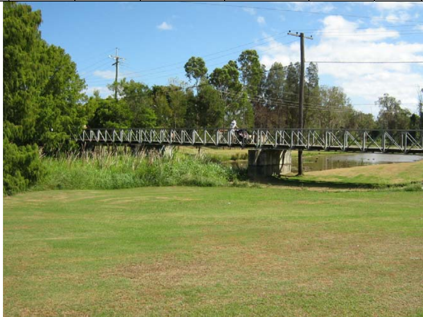
Looking downstream towards Cresswell St
