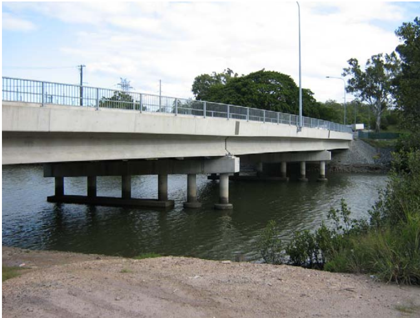
Downstream bridge looking upstream towards Gateway Motorway
