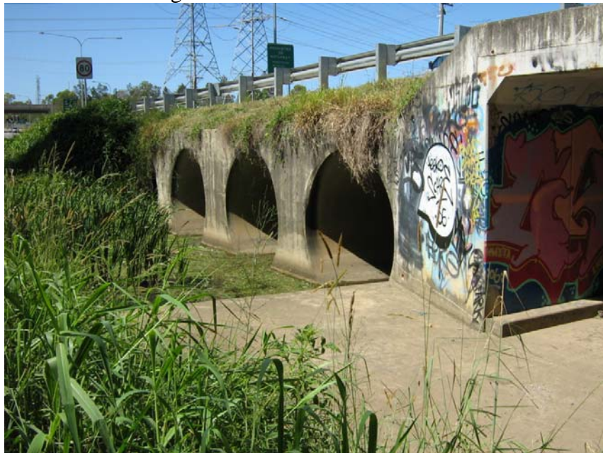
Looking upstream towards Gateway Motorway
