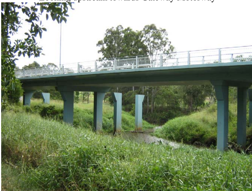
Looking downstream towards Creek Rd
