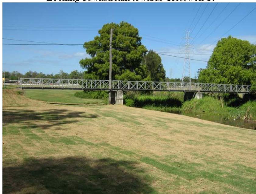
Looking upstream towards Beenleigh Road
