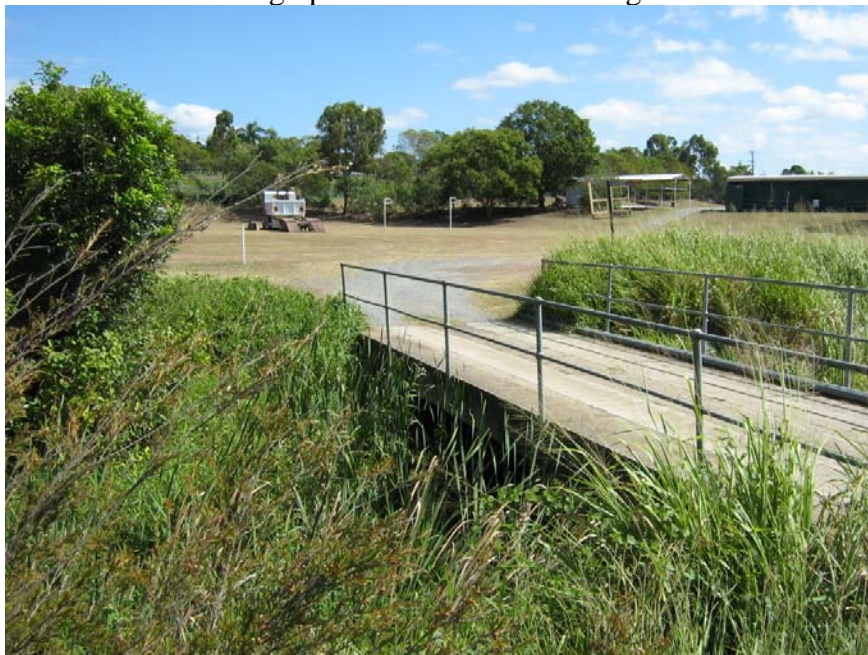
Looking downstream towards Altandi St
