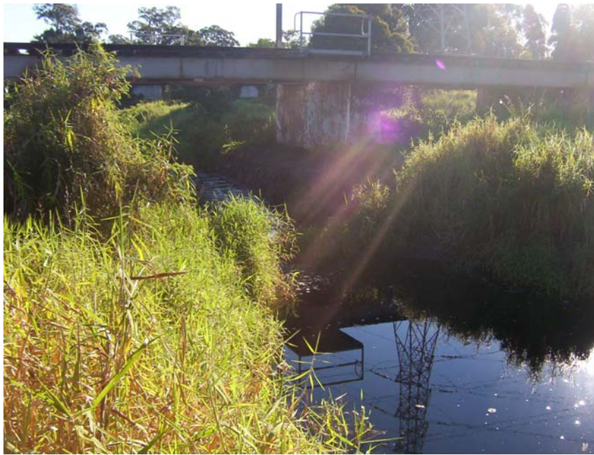
Looking upstream towards Beenleigh Rd
