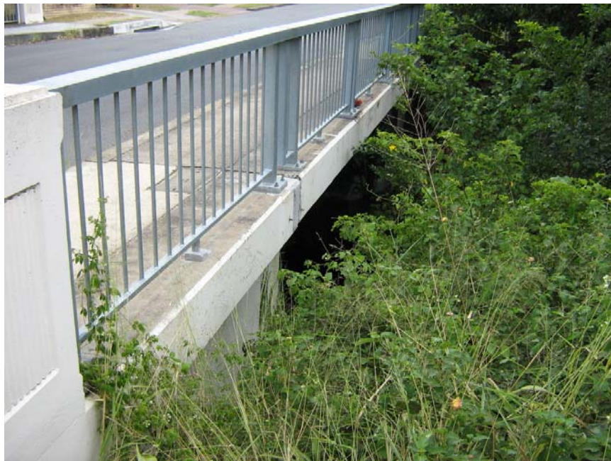
Looking downstream towards South East Freeway
